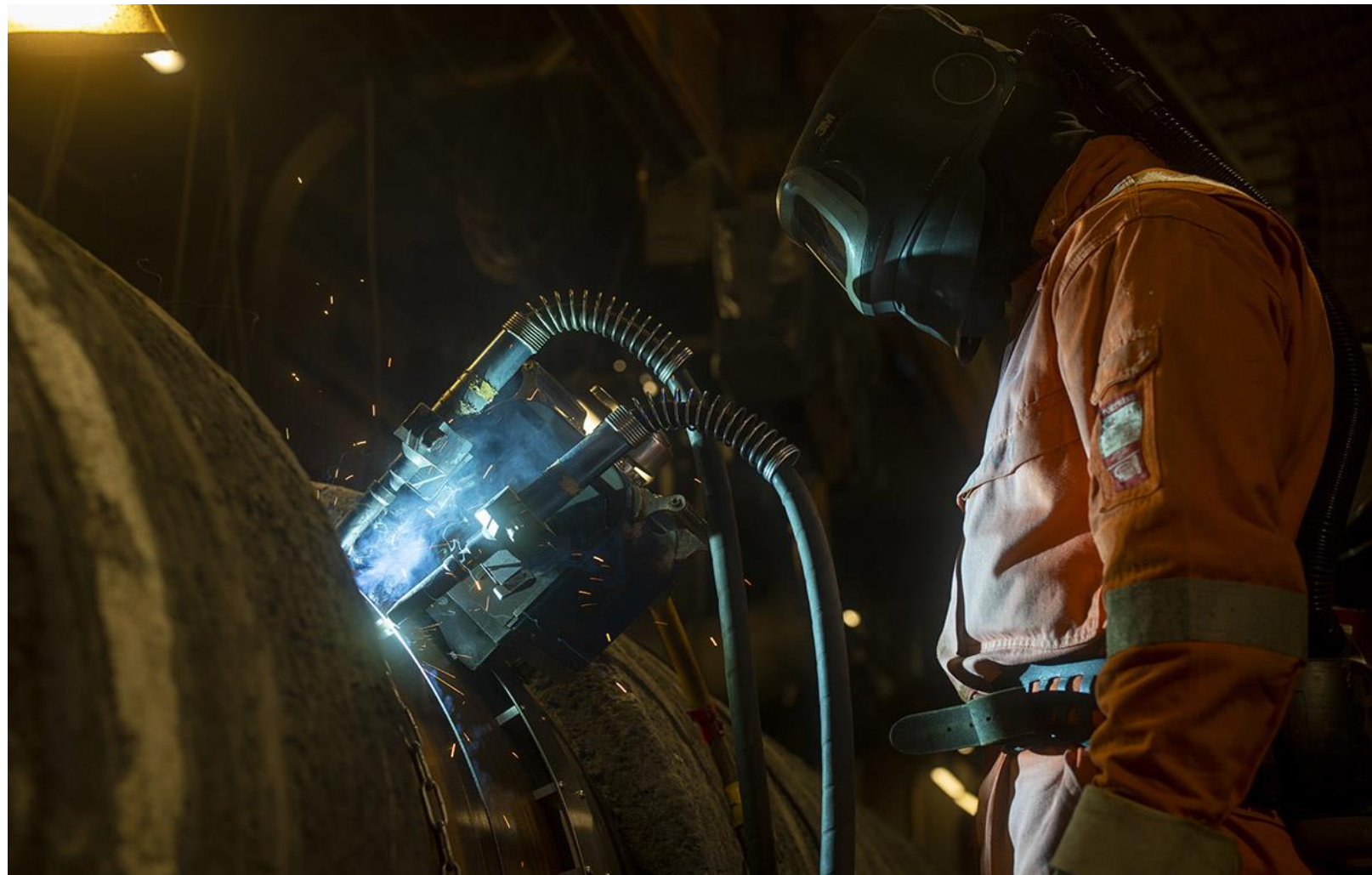
Welder on a pipelay project by Tresios Crewing Team in Baltic sea
