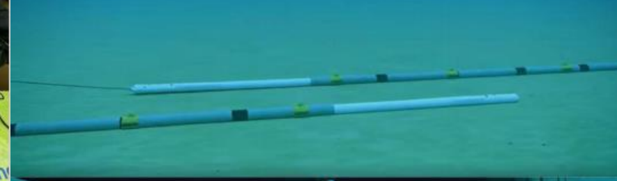
Hook-up davit lifts to 3x AWTI clamps/ pipe end
