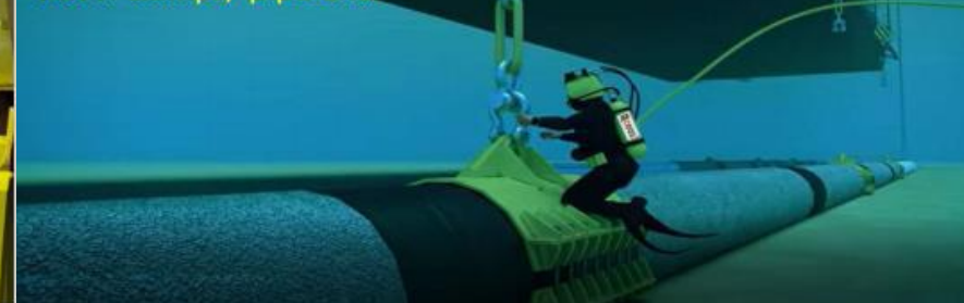
Hook-up davit lifts to 3x AWTI clamps/ pipe end
